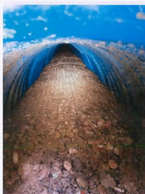
Underground stormwater detention system – replaced fully – original system was incorrectly installed, inadequate capacity.
