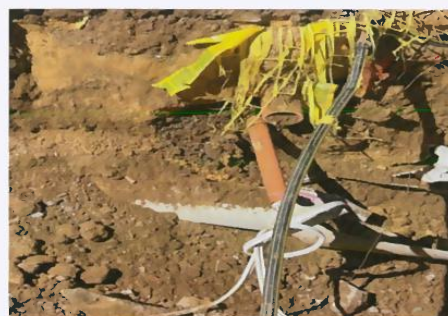
Electrical conduit showing incorrect non-standard cable
