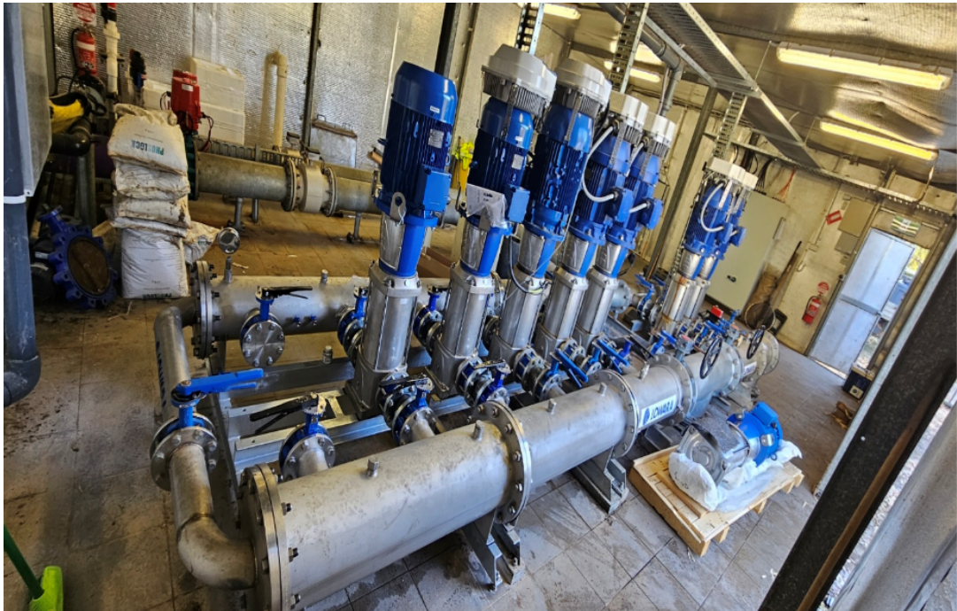
Figure 9: Pumps at the Oaklands Wetland Pump Station No 3
