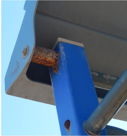
PLAY UNIT- SLIDE, DECK ETC- AT THE END OF LIFE- TO BE DEMOLISHED
