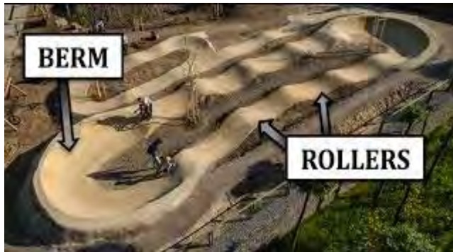
Typical tracks with compacted dirt / gravel berms as per Hallett Cove BMX track
