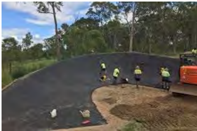
Detail showing installation of bituminized berms
