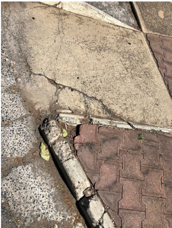
Cracked, unsafe paving along South Road, and surrounding streets of Castle Plaza.
