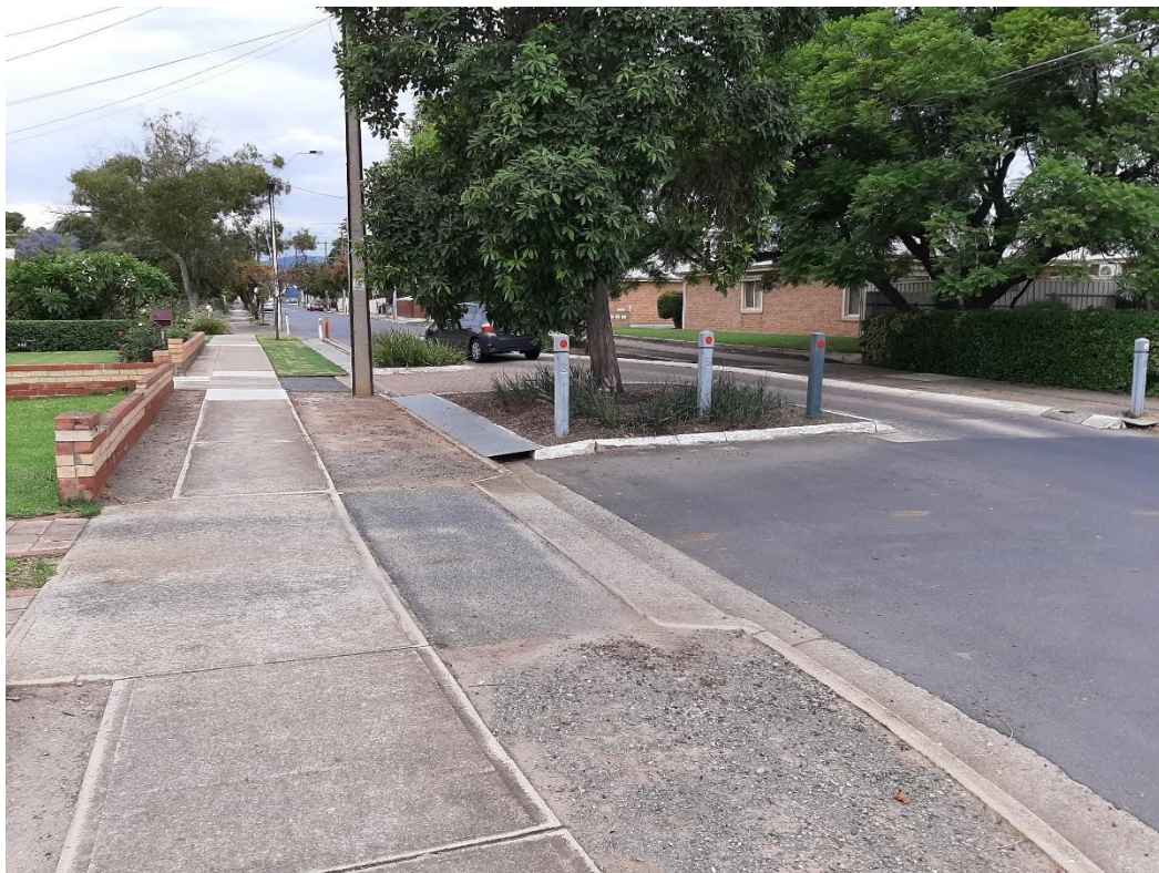
Photo 16 – post delineation on west side of driveway link
