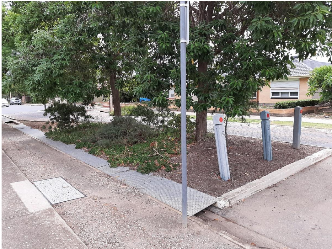
Photo 15 – post delineation on east side of driveway link, note leaning posts
