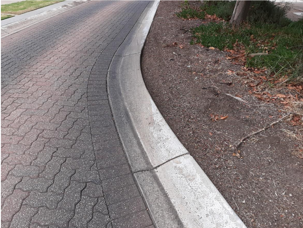
Photo 18 – kerb apex being repeatedly run over
