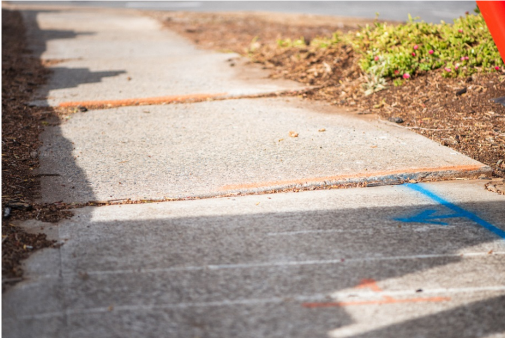
Figure 14: Tripping hazards within the footpath
