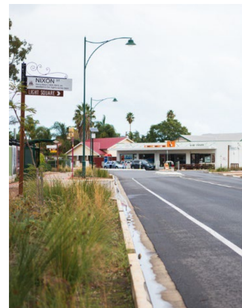
Figure 2: Kerb and Watertable located at Finnis Street, Marion
