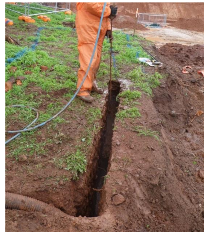
Examples of directional drilling (left) and manual excavation with hydro-excavation (right).
