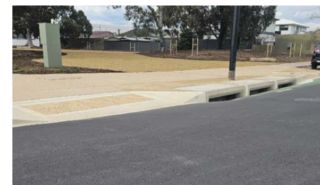
Stormwater pits
