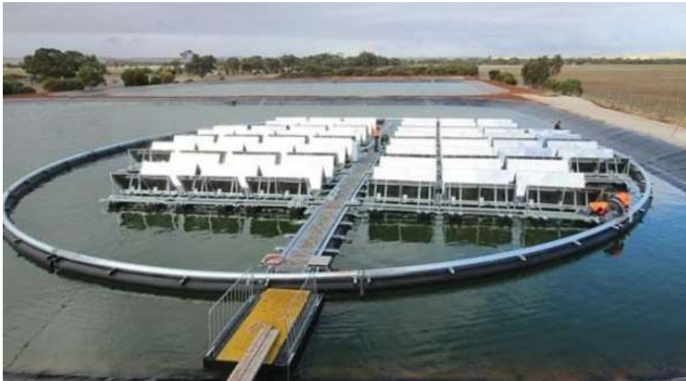
Figure 3 - Floating solar for the Jamestown wastewater treatment plant
