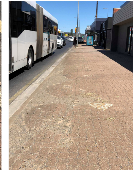
Example of how the asphalt on South Road has kicked up on to the footpath, creating an uneven and unsafe space.
