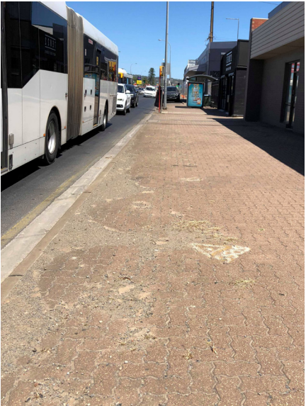
Example of how the asphalt on South Road has kicked up on to the footpath, creating an uneven and unsafe space.
