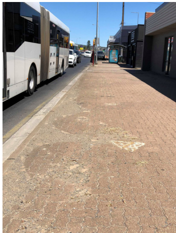
The asphalt on South Road has kicked up on to the footpath, creating an uneven and unsafe space.
