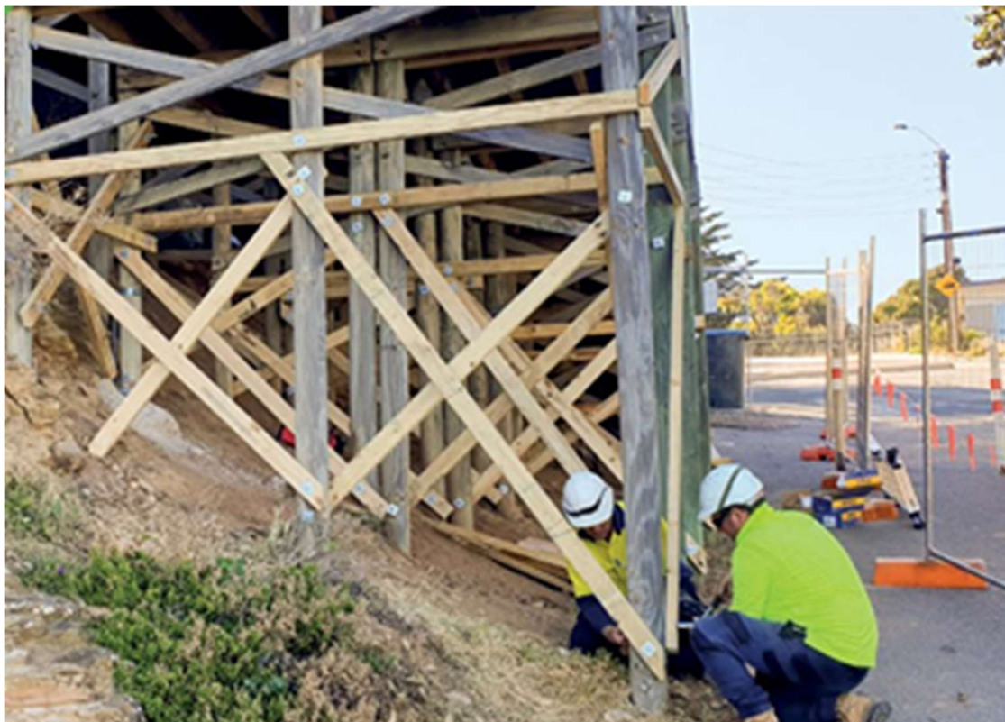
Figure 13: Repairs to Coastal Walkway structure
