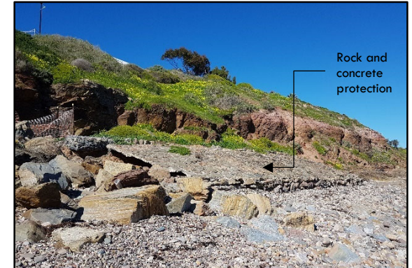
Figure c. Rock and concrete sloping seawall protected former building in this location (see aerial photograph, 1979).
