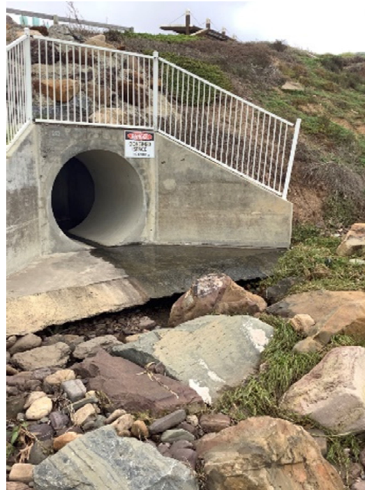
Figure (a) Outlet 3.1. Under the concrete base has been eroded away in recent storm events. Suggest fill.
