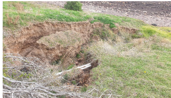
Figures (a) and (b). The storm water infrastructure was likely under engineered in the first instance due to the remote location. The pipes have broken, and gully formed from storm water flows from Balboa Drive.
