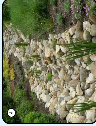
Item J - Native revegetation & enhancement of existing stormwater rock swales
